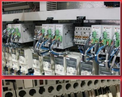
The Ultra-fast Techna-Check transducers are developed specifically for Machine Tool Monitoring applications and can monitor both AC and DC loads. These sensors mount in the electrical cabinet of the machine and communicate with the Techna-Check units using the proprietary TTBUS network.
